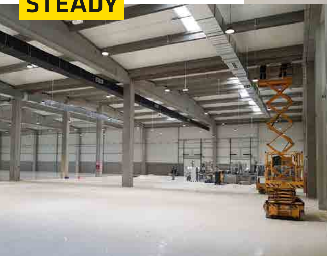
Production is about to start in Romania
